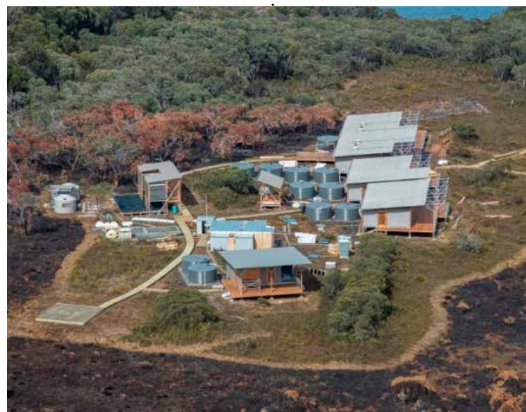
A hut on the Three Capes Track. Similar huts are planned along the South Coast Track, below Federation Peak and at the Walls of Jerusalem.
