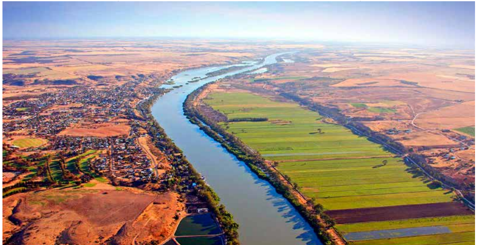
Aerial of Mannum on the Murray River, South Australia. Photo: S. Strudwick
