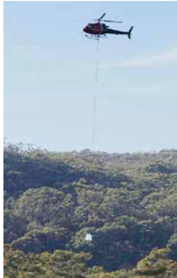
The NPWS used Bulka bags to chopper in sandstone blocks and materials for mountain bike track construction in Garigal National Park and to remove huge amounts of native vegetation after due process. For Royal National Park, due process may reward the builders of illegal MTB tracks. Photo: H. Gold
