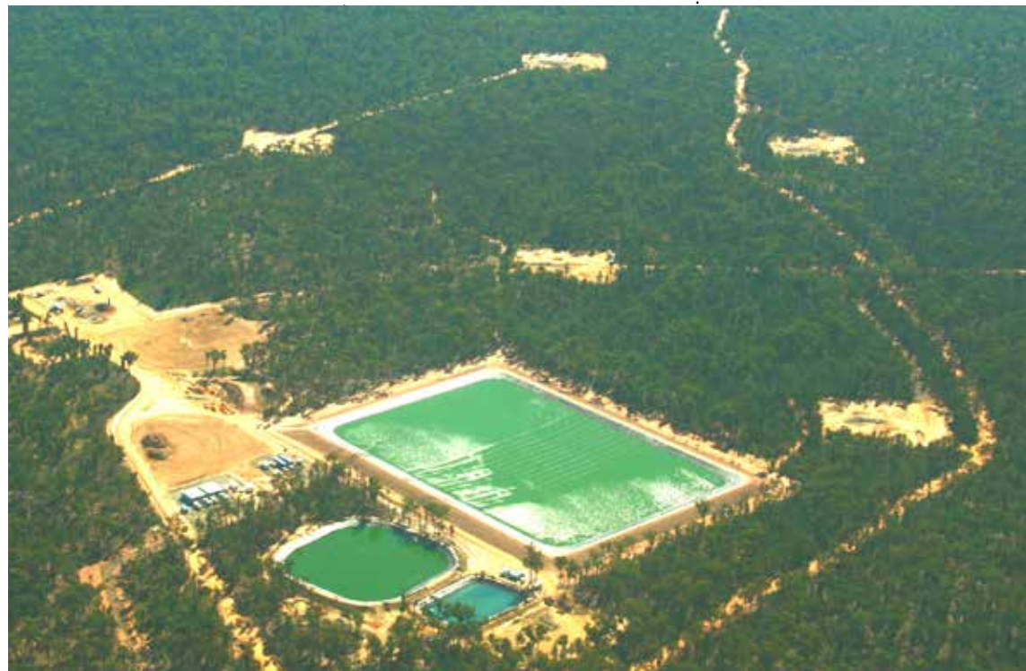
Storage of produced water from earlier CSG gas mining in Bibblewindi State Forest.
