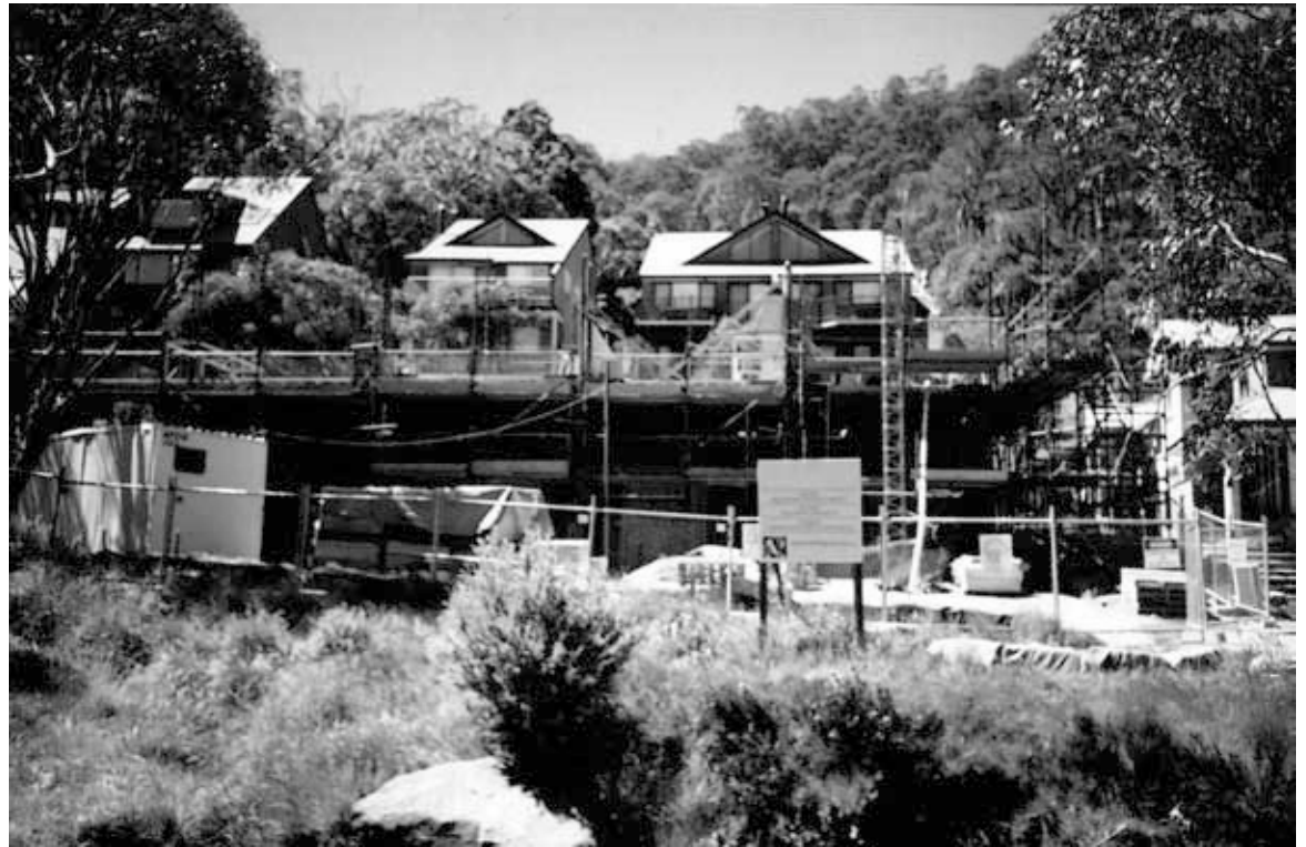
The cutting of red tape proposed by the State Plan review could make park development much easier, such as that this recent development at Thredbo in Kosciuszko National Park.
